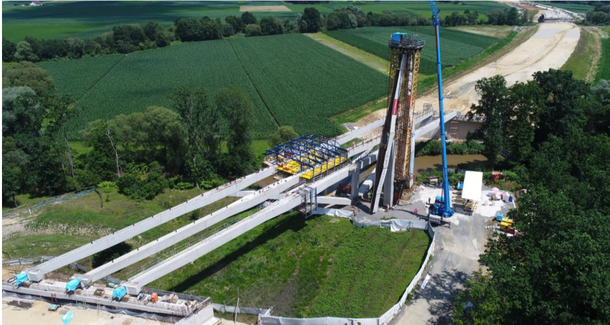
▲ Construction of Lafnitz bridge on the S7 motorway in Austria
