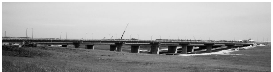
Bild 1. Floodway Bridge in Winnipeg Manitoba (Photo: Fortius)
